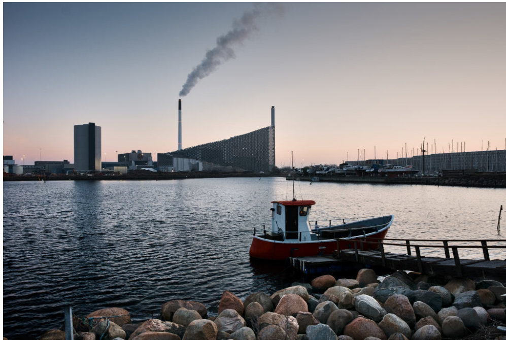
Amager Bakke Energy Plant, a combined heat and power waste-to-energy plant in Copenhagen, Denmark. Photo credit: Amager Resource Center.
