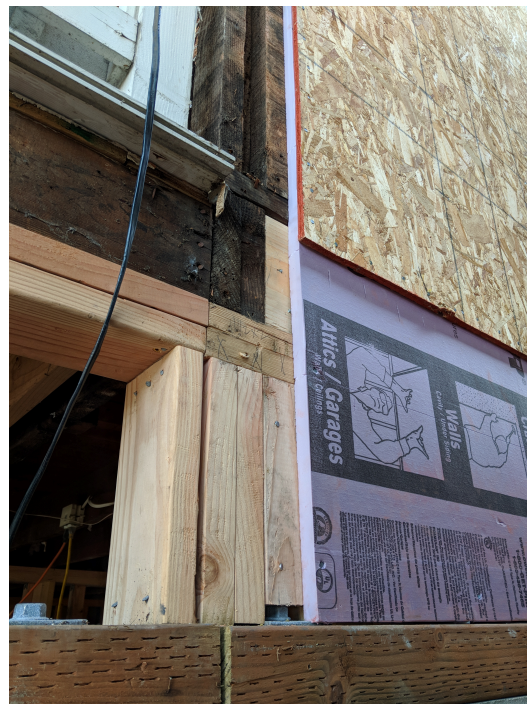
Figure 8: TBS wall layers on old and new wood studs
