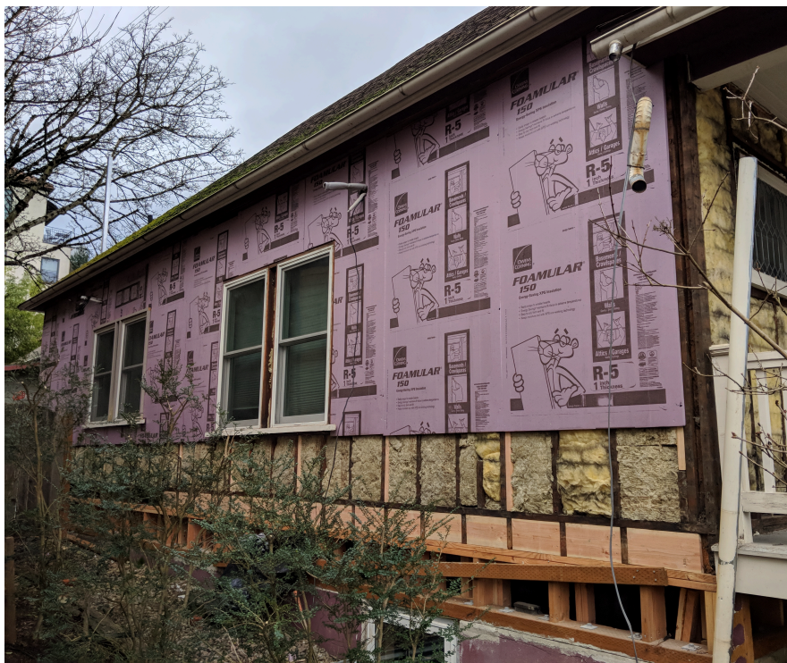
Figure 5: Rigid foam installation
