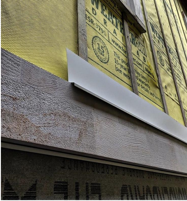
Figure 11: Weather-resistant barrier, rainscreen, and flashing
