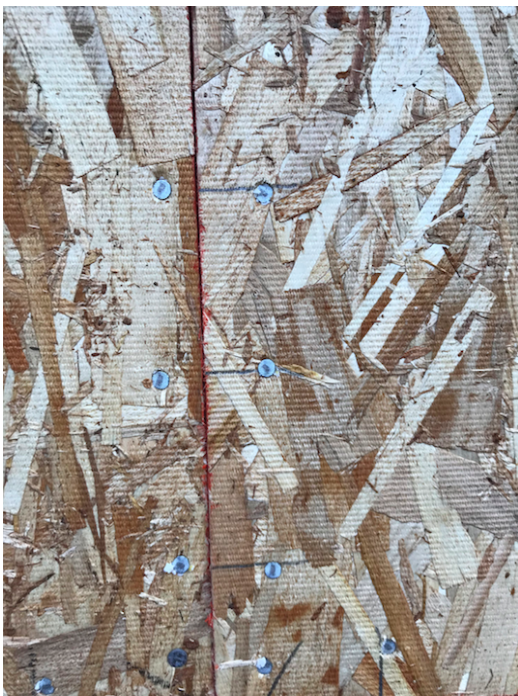
Figure 7: Specific nailing pattern
