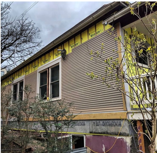
Figure 12: New siding installation
