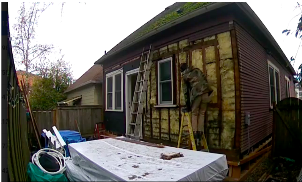
Figure 3: Siding removal
