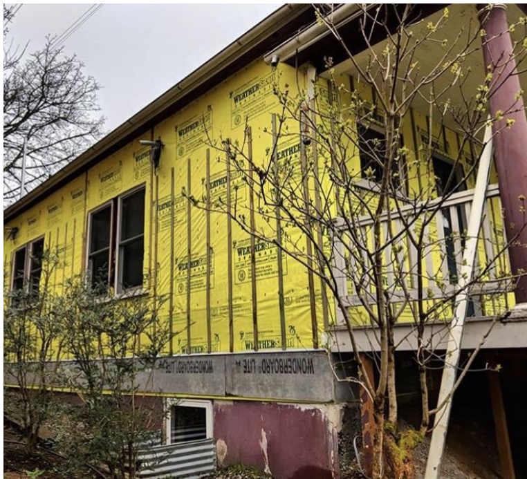
Figure 10: Weather-resistant barrier and rain screen
