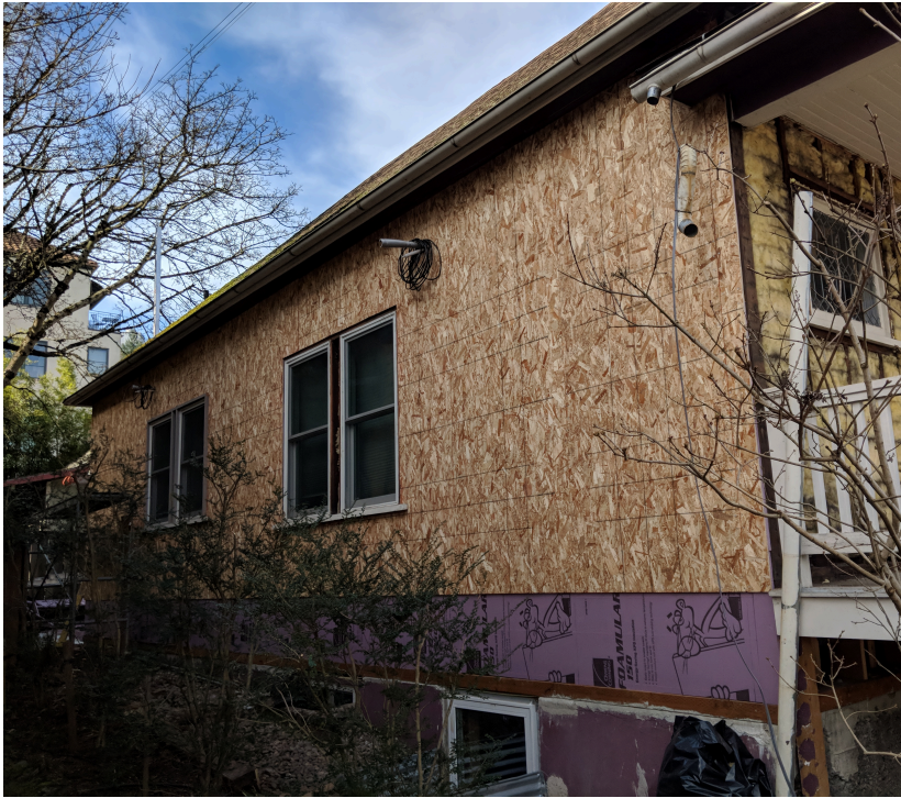
Figure 6: Sheathing installation
