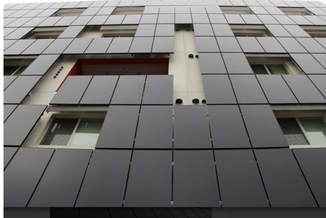
Figure 60: Residential building facade in Los Angeles overclad with mono-crystalline PV modules © KoningEizenberg
