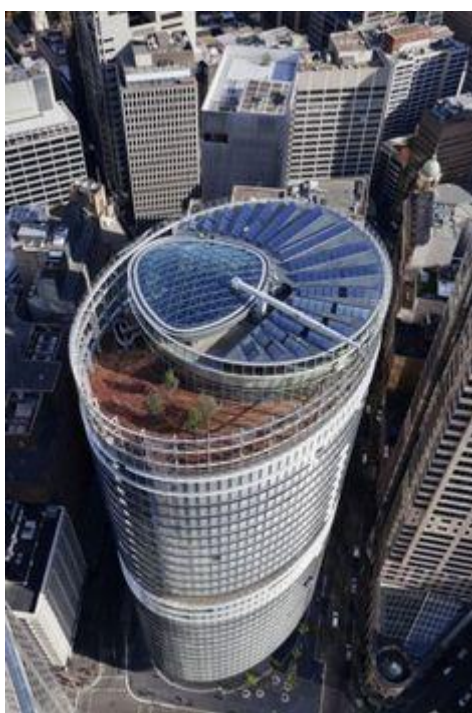
Figure 57: Aesthetically arranged solar thermal array on roof of 1 Bligh Street, Sydney
