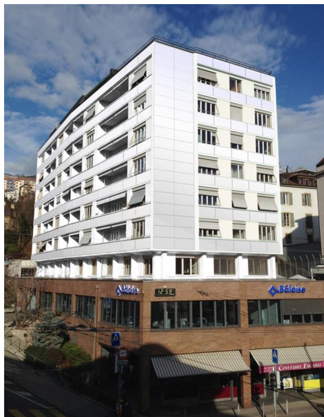
Figure 61: Commercial building clad in pioneering white PV modules, Neuchâtel, Switzerland © Solaxess
