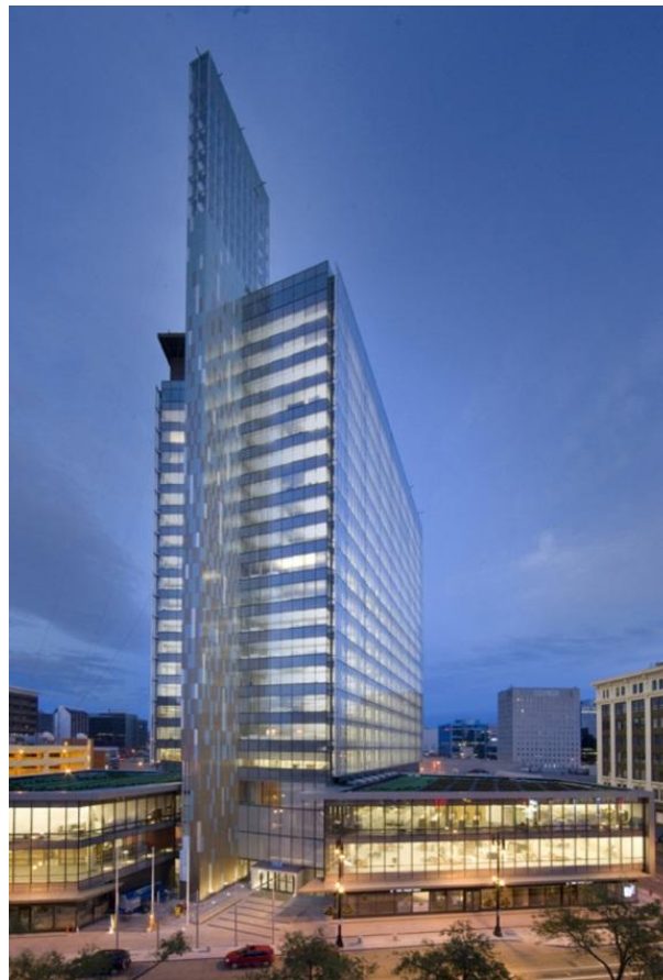
Figure 43: 115m high solar chimney providing passive ventilation whilst making an iconic design statement
