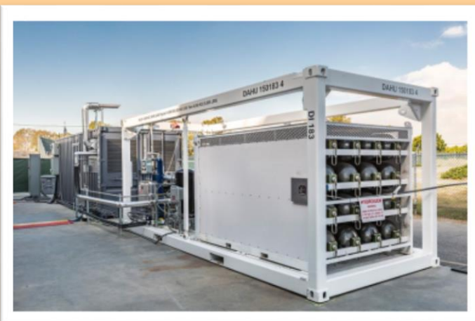
Figure 2.32: Picture of a Sunfire SOEC unit (from https://hydrogeneurope.eu/member/sunfire )
