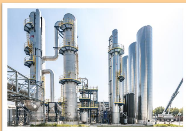
Figure 2.4: Amine absorption plant for carbon capture on waste incineration plant at AVR in Duiven, The Netherlands. Photo: NIRAS A/S
