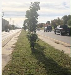
Medians often present a harsh environment for vegetation, given their high exposure to road salt. To increase infiltration, reduce maintenance, and increase vegetative growth, the project team replaced the existing crowned, compacted soil with a compost/biochar mix.
