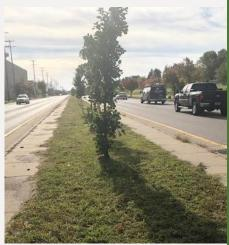
infiltration. Medians often present a harsh environment for vegetation, given their high exposure to road salt. To increase infiltration, reduce maintenance, and increase vegetative growth, the project team replaced the existing crowned, compacted soil with a compost/biochar mix.
